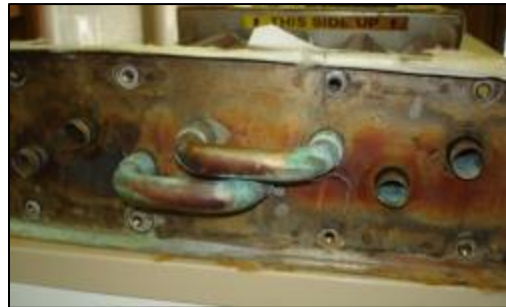
Sooted – Improper Fuel and Air Mixture.
